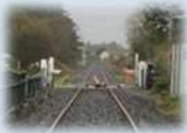
On the 23<sup>rd</sup> October, as a train was travelling in damp weather, the train began to experience LRA conditions, resulting in the driver not being able to fully control the train causing the train overrunning Ardrahan Station Platform, passing a signal at danger and travelling through a Level Crossing XE156 with the barriers raised to road traffic.
