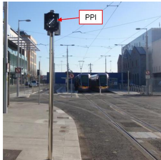
Photograph 2 – Tram signal at facing points
