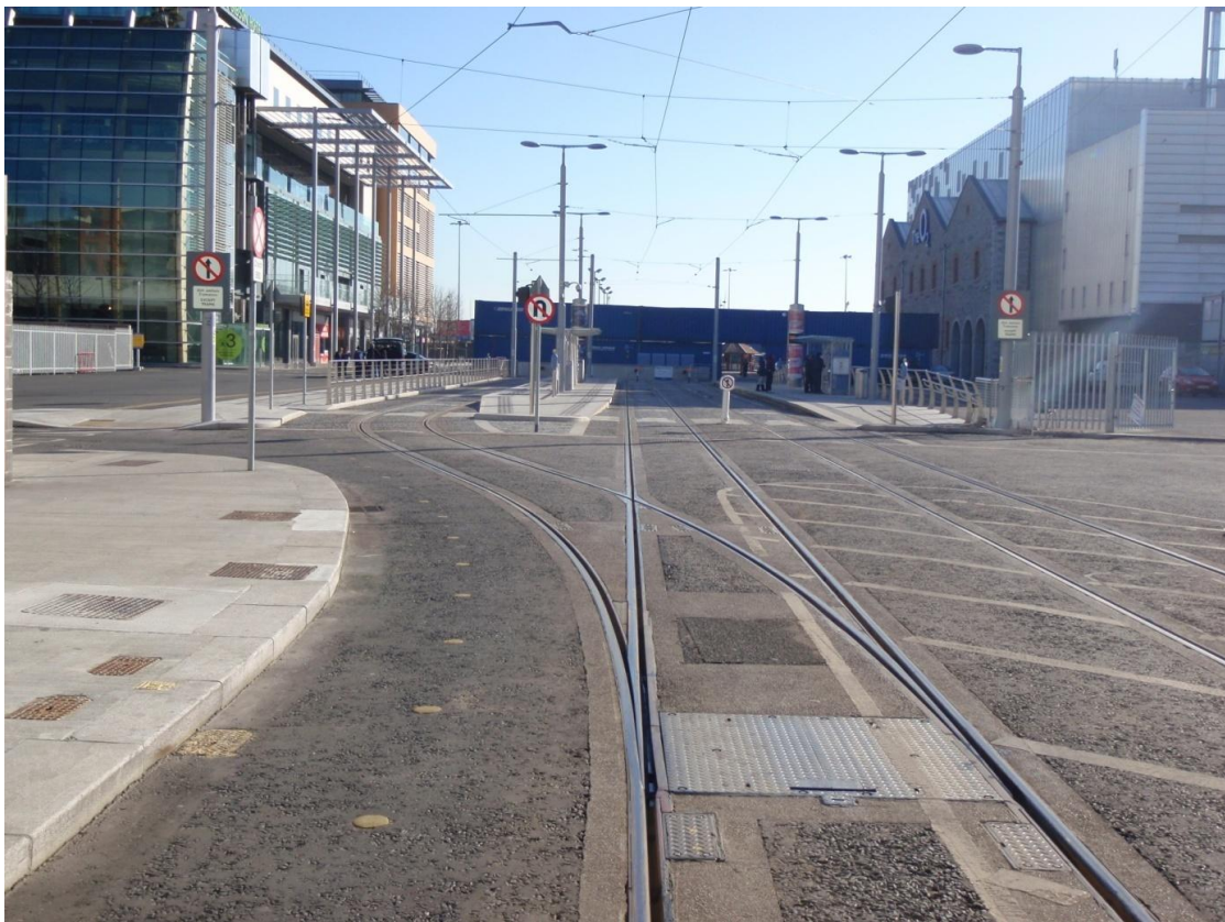
Tram derailment at The Point Stop, Luas Red Line
