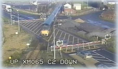
At approximately 11:10:56 hrs, the 09:45 hrs passenger service from Westport to Heuston (Train A805) triggered the initiation for Level Crossing XM065 (a CCTV level crossing with lights and full barriers), which resulted in the road traffic lights flashing to indicate to road users that rail traffic was approaching. Two cars approached the level crossing from the Athlone direction, after this initiation had commenced, with one car stopping on the yellow box area (Car 1),
