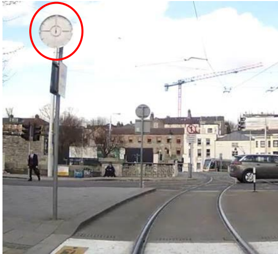
Figure 6 – Missing mirror
