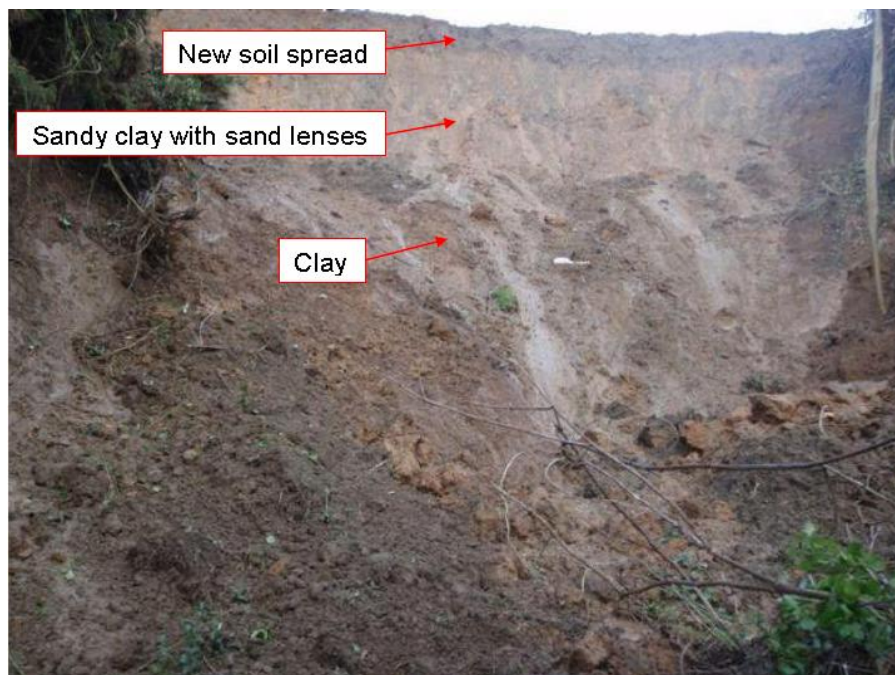
Photograph 2 – Cutting geotechnical properties
