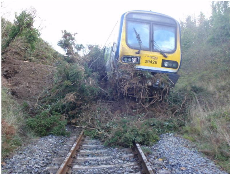
Photograph 1 – Derailed train on landslip debris
