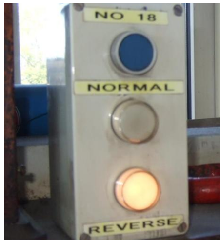
Photo 4 – Turnout direction release button
