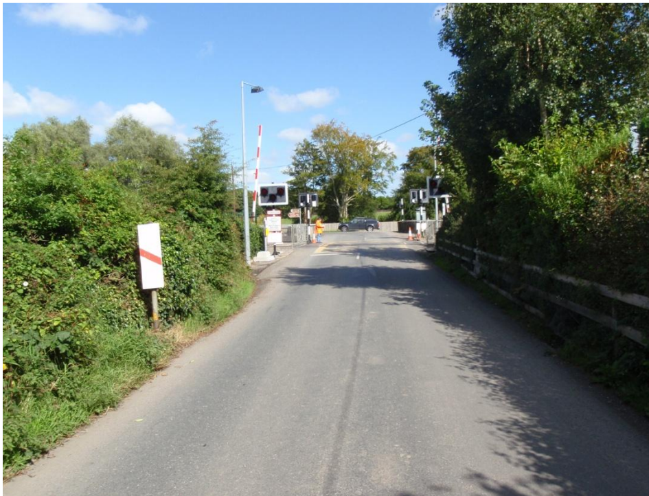
Photograph 5 – Approach to Ferns Lock AHB
