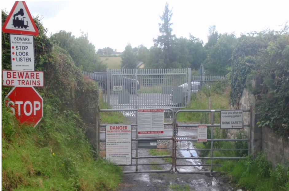
Figure 5 – Up side level crossing approach
