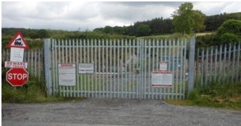
Figure 4 – Down side level crossing approach
