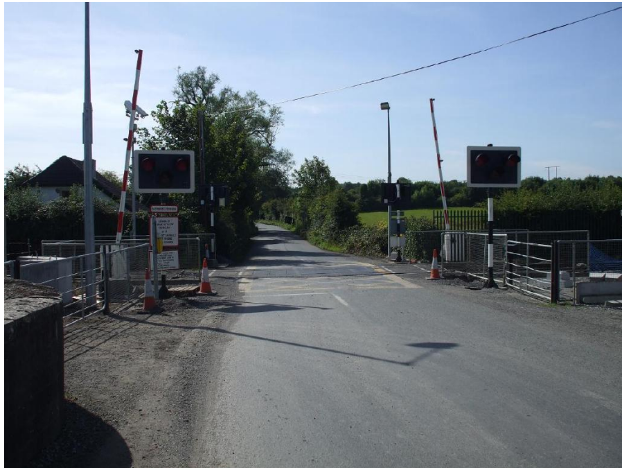
Photograph 4 – Ferns Lock Automatic Half Barrier
